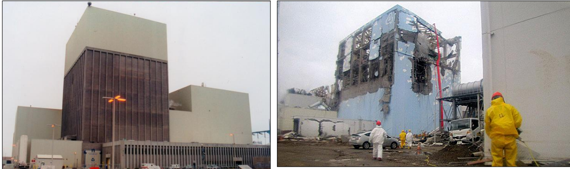
Side-by-side comparisons of the GE boiling water nuclear reactors at the Columbia Generating Station (left) and at Fukushima (right) reveal a similar design. Photos courtesy of CLUI (left) and Fukushima Update (right).
