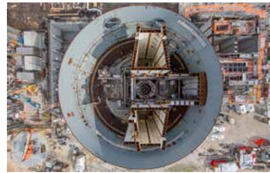
The Vogtle #4 reactor under construction in Georgia.
